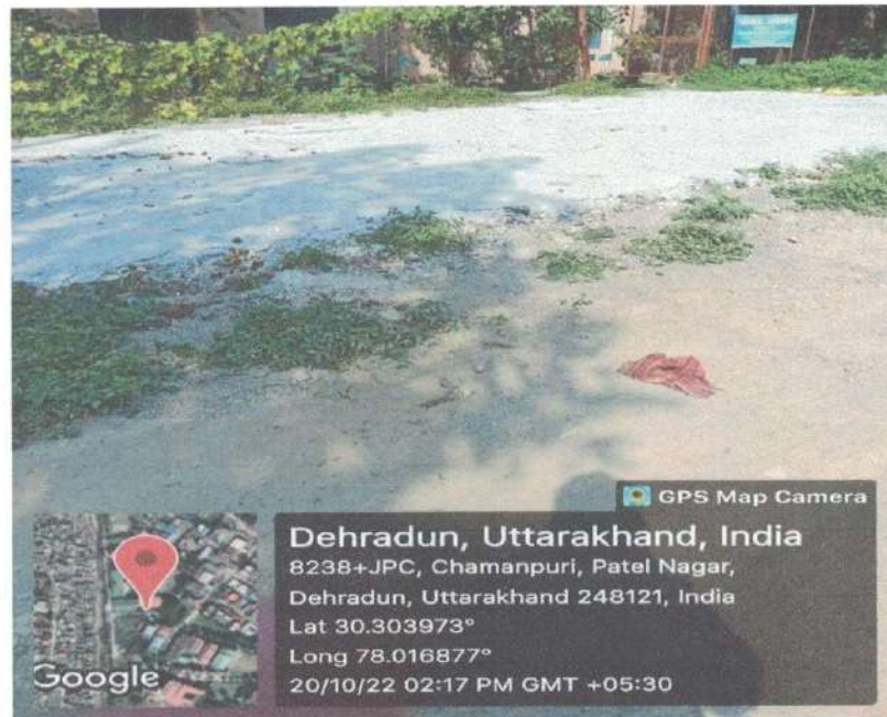
Fig-4.6: Rain Water Harvesting Pits in the University
