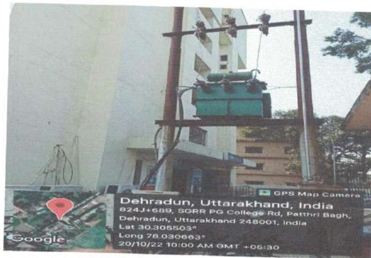
Fig-3.8:11/0.4 KV Sub station, S.G.R.R University, Pathribagh
